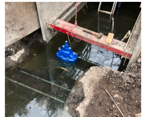
The existing main was underneath the water table, so continuous pumping was necessary to be able to conduct the weld and perform the hot tapping. The Plasson Large Bore Saddle was installed with minimal digging and lightweight equipment.
